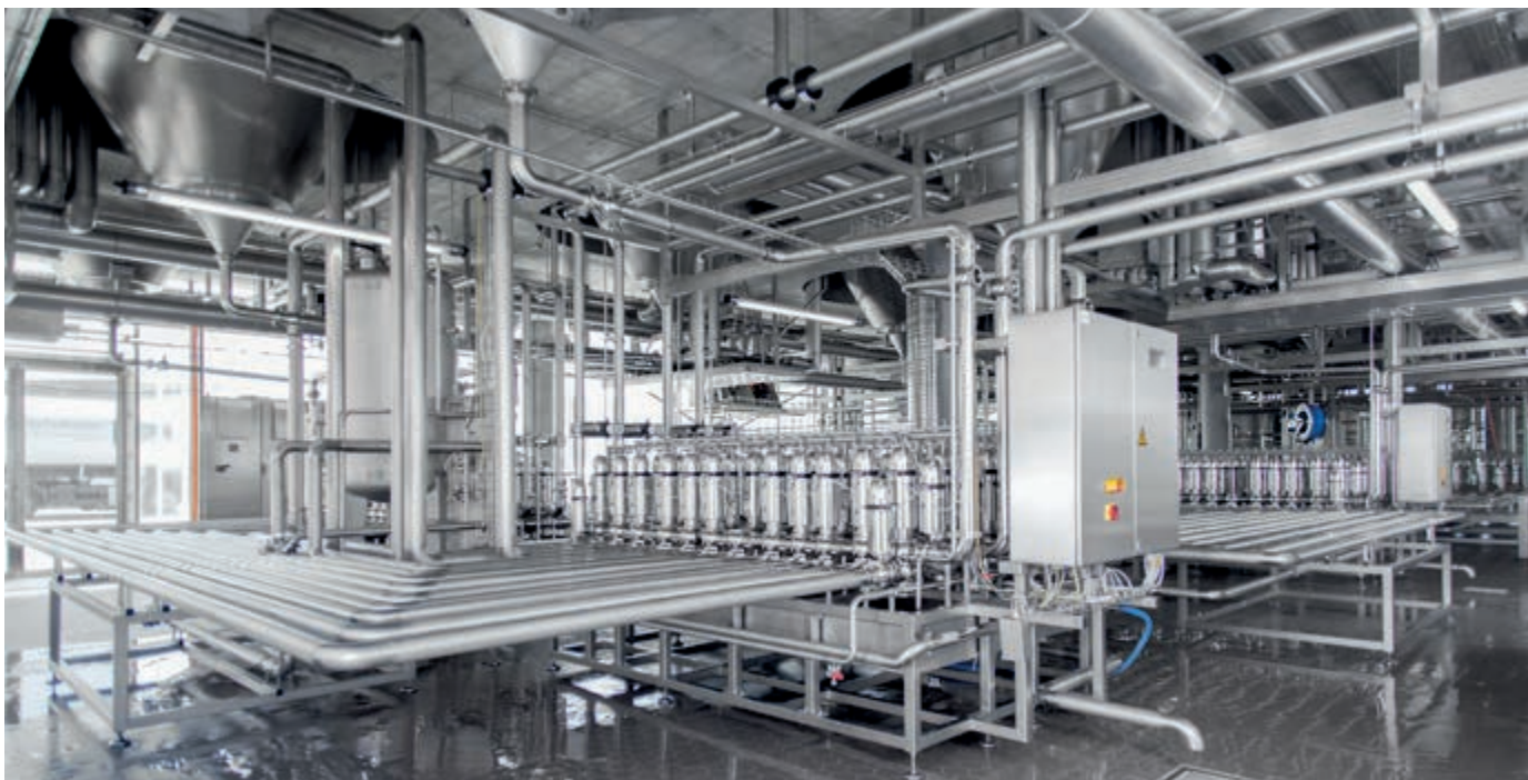
4,000 metres of carrier tube and 5,400 metres of beverage line tube (900 metres of which are pre-insulated) for a state-of-the-art fermentation and storage cellar
